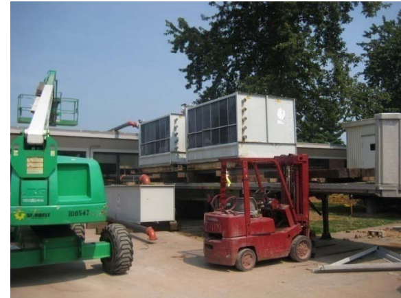
Relocation of Chiller
