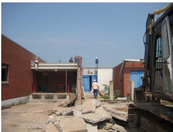
Demo of Existing Mechanical Room
