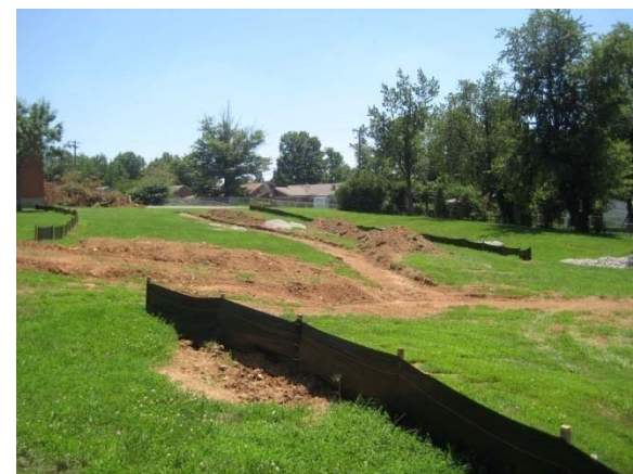
Site Demo for New Sidewalks
