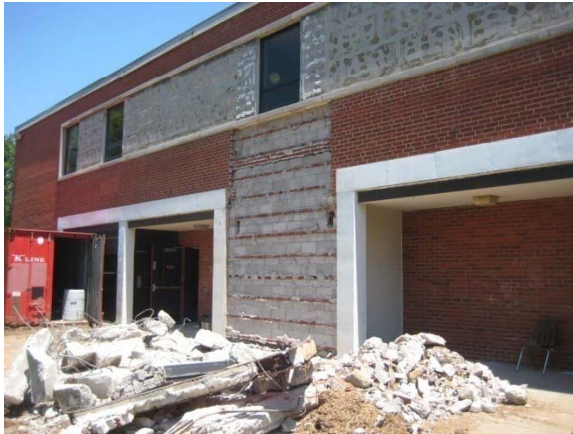
Demo of Existing Structure
