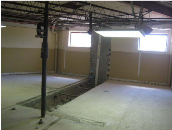
Demo of Restrooms
