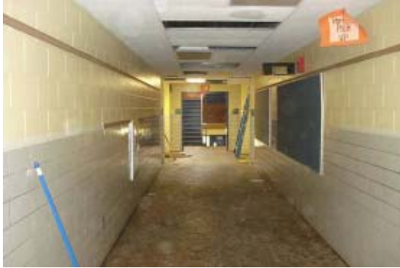
Abatement of Corridor
