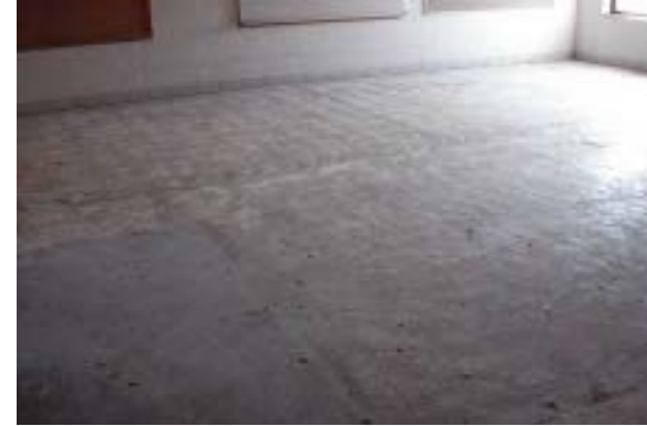
Removal of Tile
