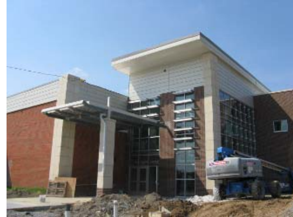
Exterior Glazing Work
