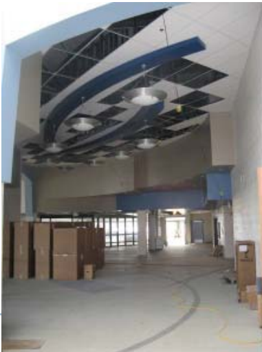
Lobby -- Terrazzo Floors & New Ceiling
