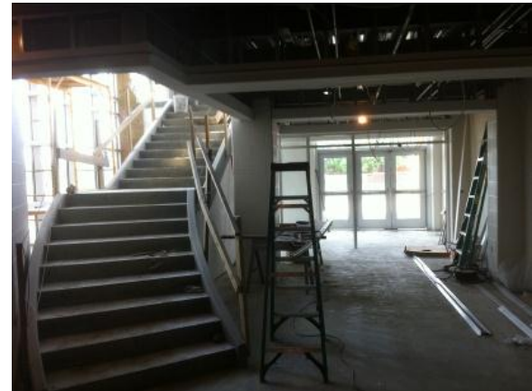
Handrails at New Stair
