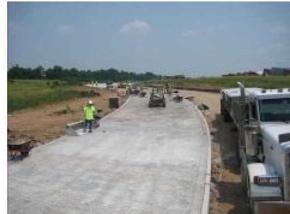
Pervious Pavement on Main Entry
