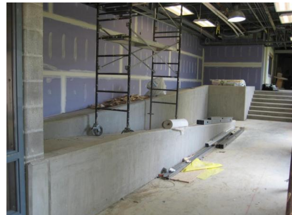
Corridor Handicap Ramp
