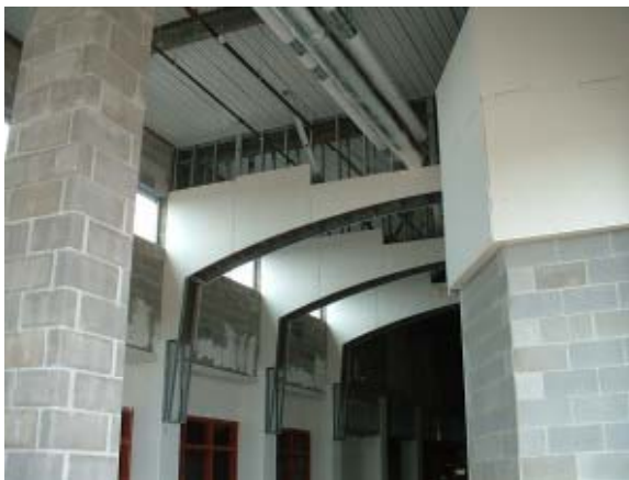
Metal Framing of Soffits
