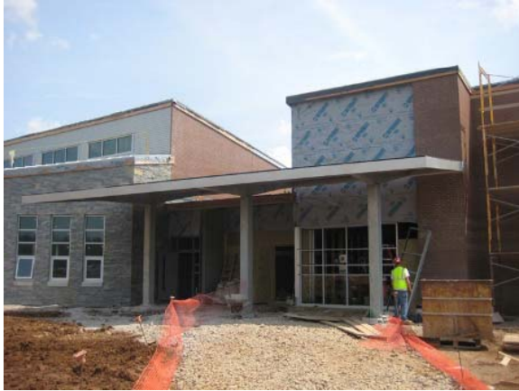
Academic Bldg.—Entry w/ Green Roof Structure
