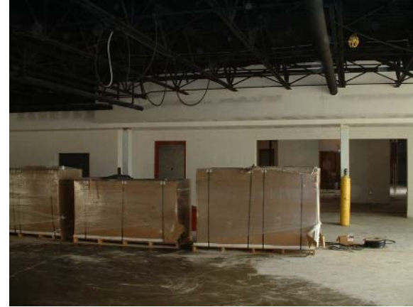
Installation of Kitchen Equipment
