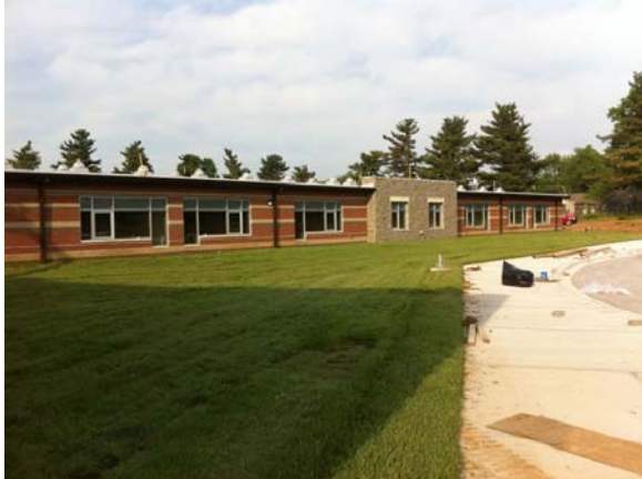
Sod is Being Installed
