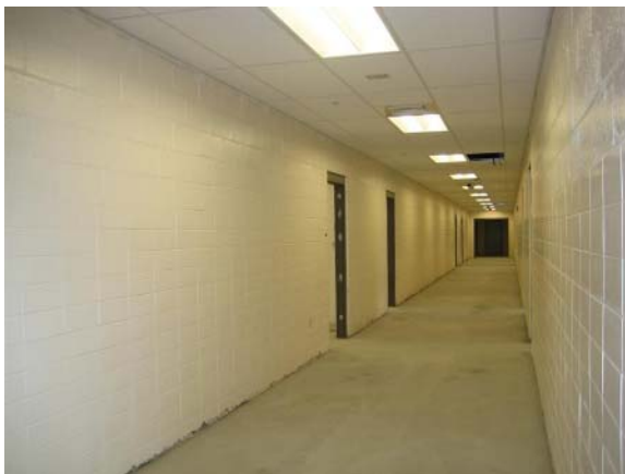
Area "C" Corridor
