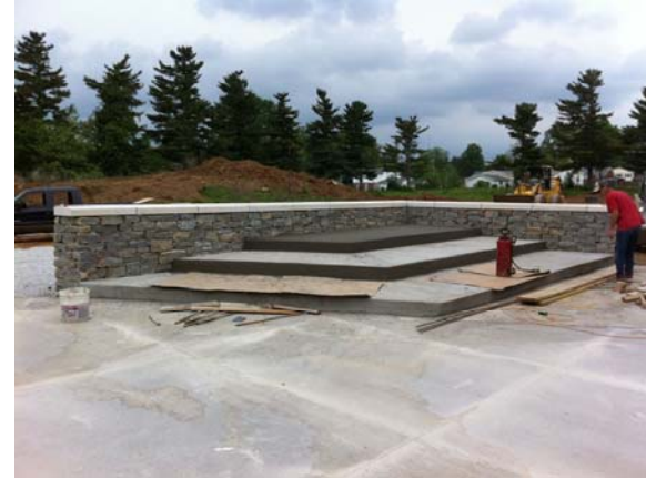
Concrete Landings – Outdoor Classroom
