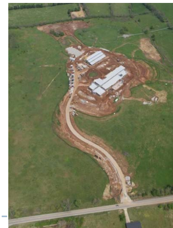
Aerial Site View
