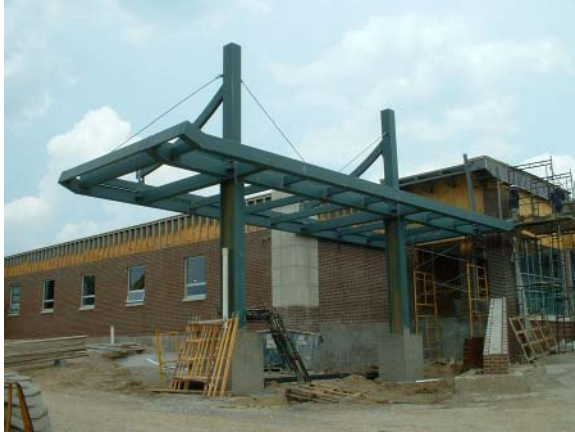
Structural Steel on Canopies
