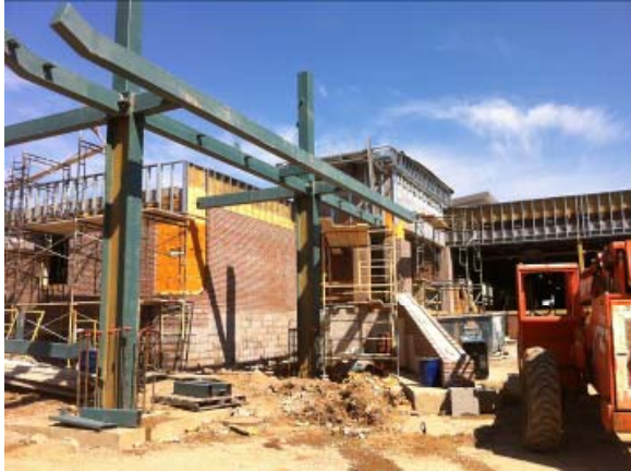
Structural Steel on Canopies
