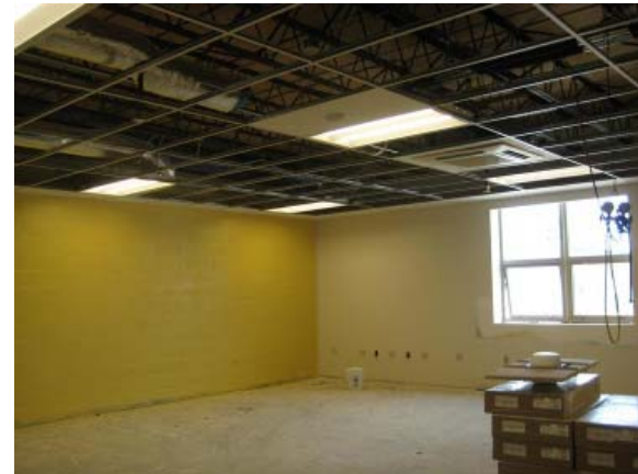
Area "C" Classroom—Finishes
