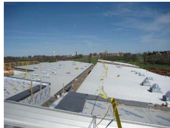
Academic Bldg.—Standing Seam w/ Solatubes
