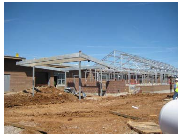
Store & Greenhouse Framing
