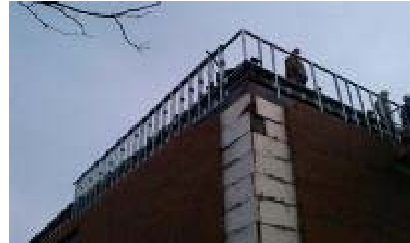
Parapet Wall Surround
