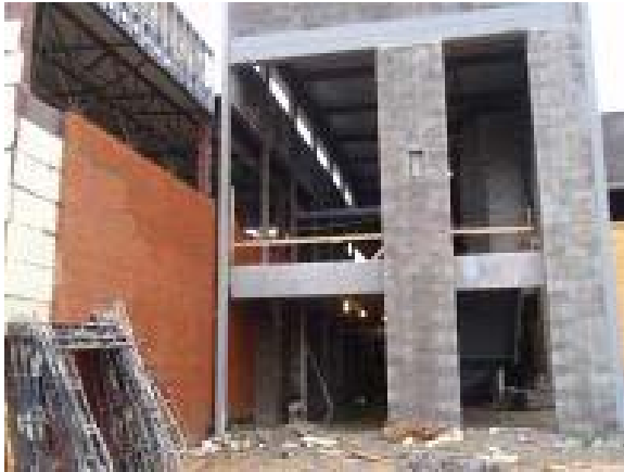
Metal Roof Decking
