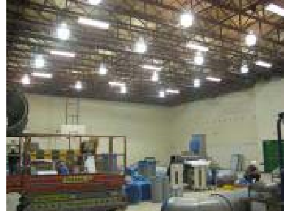
Gym—Demo & New Lights
