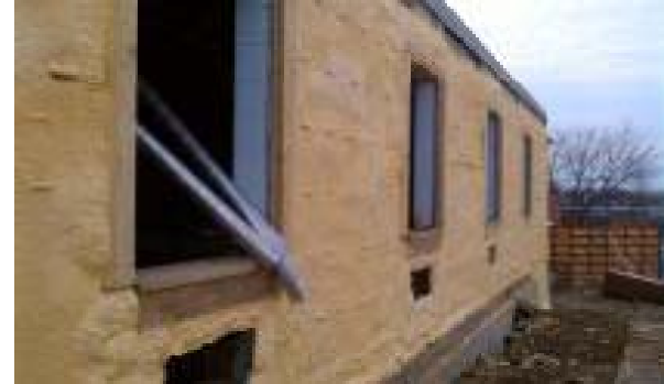
Foam Insulation—Exterior Walls
