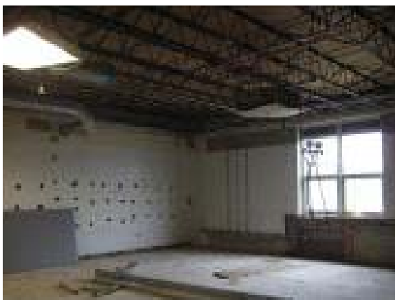
Area "C" Classroom -- Demo
