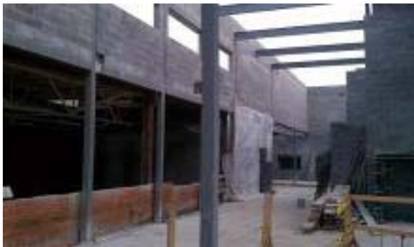
Phase I Steel Structure
