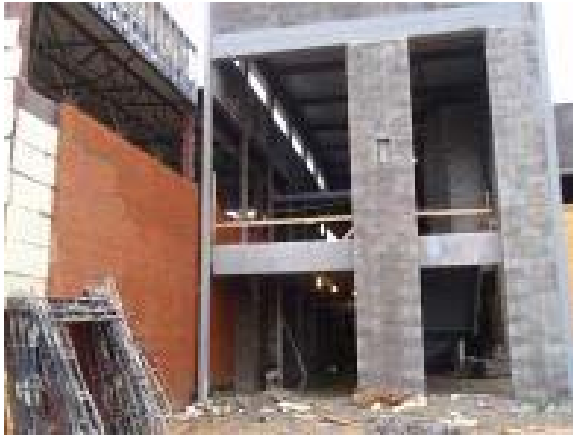
Metal Roof Decking
