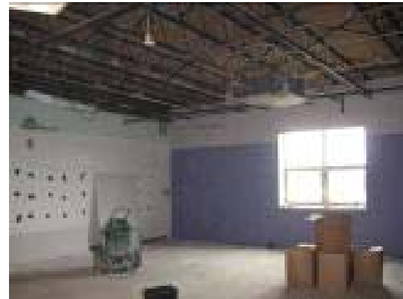
Area "C" Classroom—New Exterior Wall
