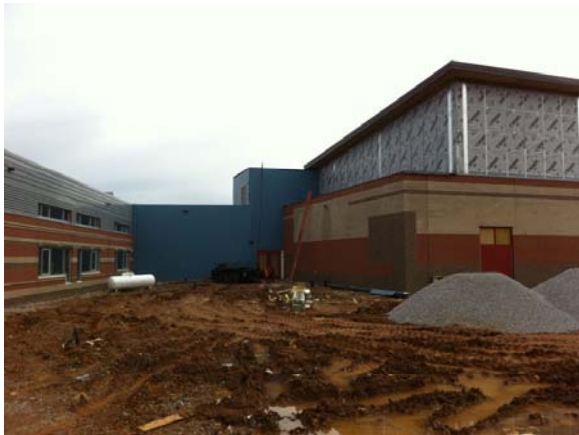
Metal Wall Panel Installation
