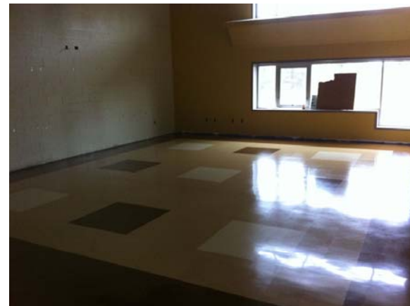
Floor Tile Installation
