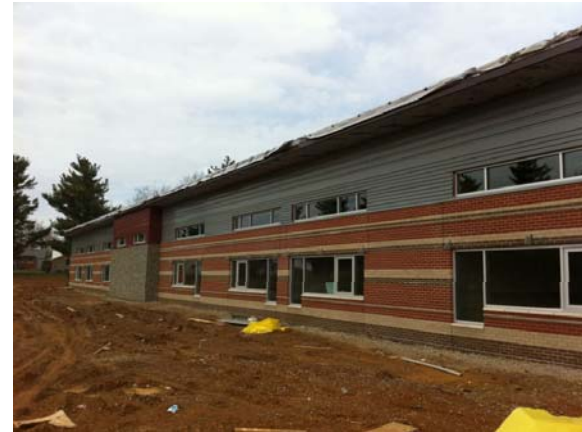
Metal Wall Panel Installation
