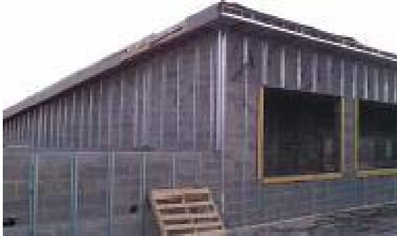
Framing & Roofing in Courtyard
