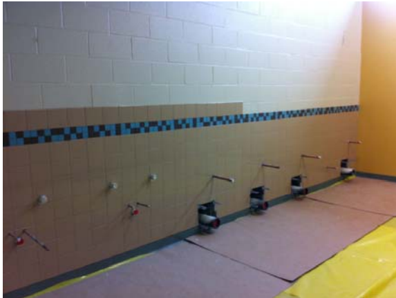
Tile in Restrooms
