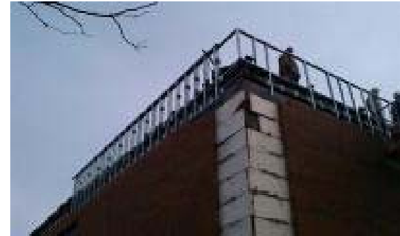
Parapet Wall Surround
