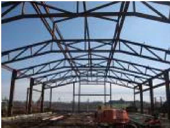
Riding Arena—Roof Structure
