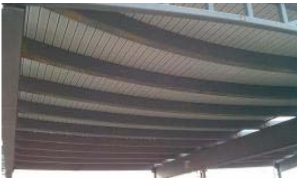
Media Ctr. Acoustical Roof Deck
