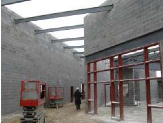
New Main Corridor
