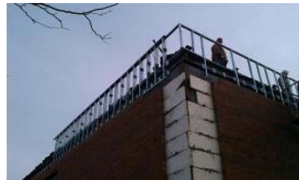
New Roof Parapet
