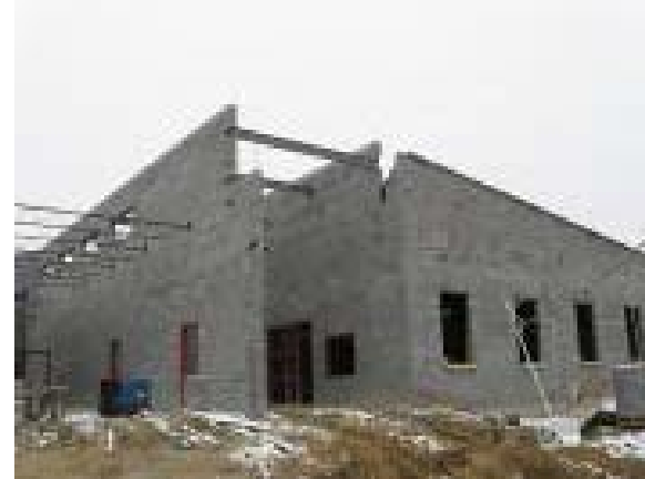
CMU at New Entrance
