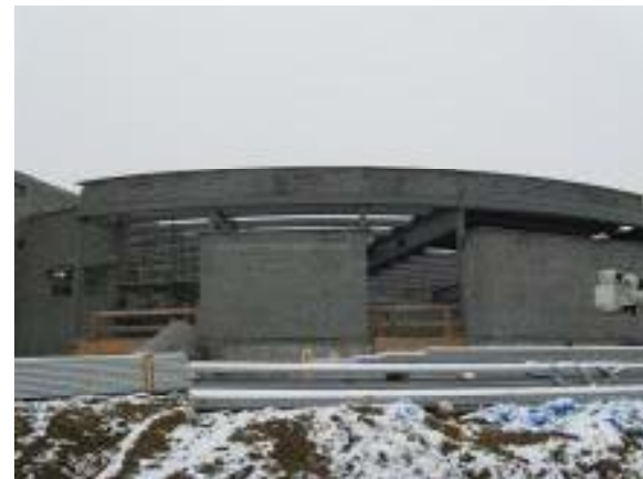
CMU Walls at Media Ctr.
