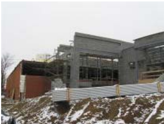
CMU Walls at Gym
