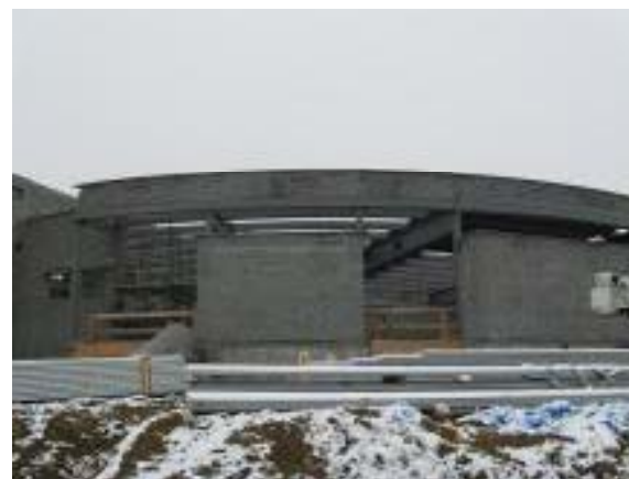
CMU Walls at Media Ctr.
