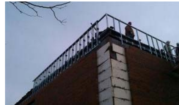
New Roof Parapet
