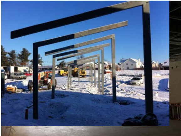
Entry Canopy Installation
