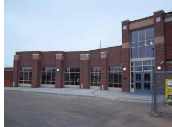
Main Entry - Admin. Area
