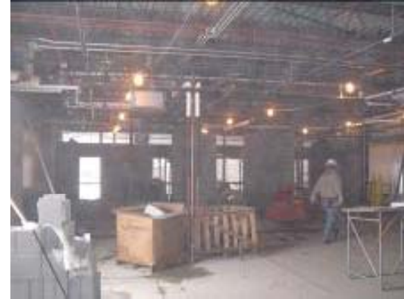
Mechanical & Plumbing Rough-ins
