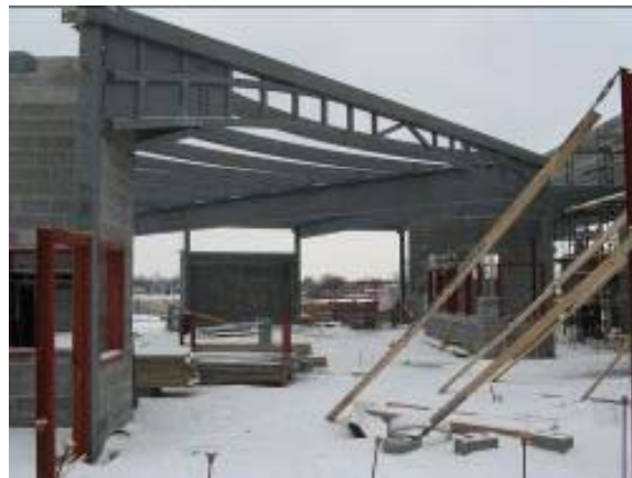
Metal Framing around Courtyard
