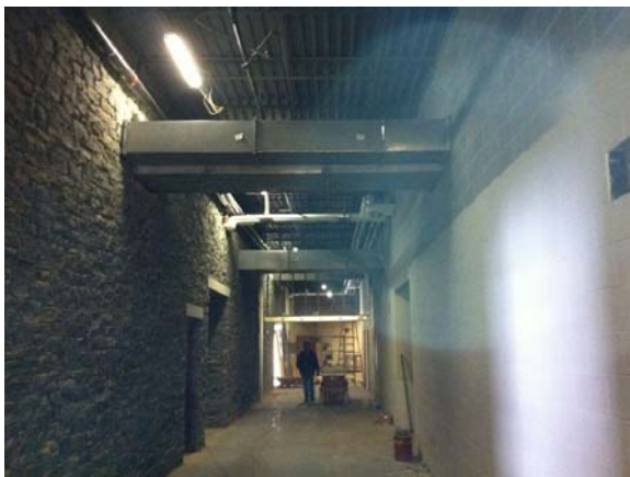
Ductwork Installation
