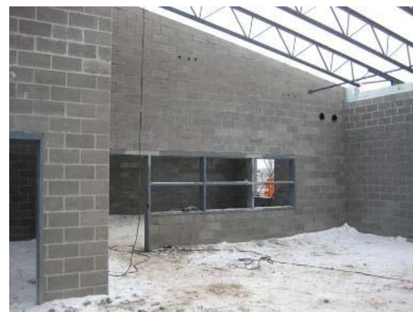
Academic Bldg. – Typical Classroom from Lab
