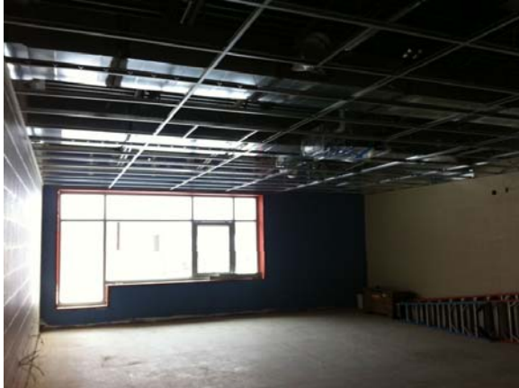
Ceiling Grid Installation
