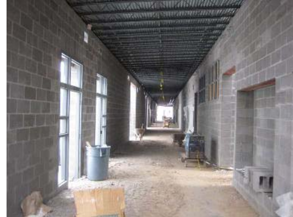
Academic Bldg. – Main Corridor
