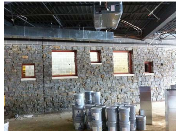
Interior Precast Window Sills
