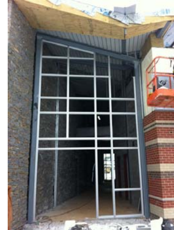
Curtainwall Installation
