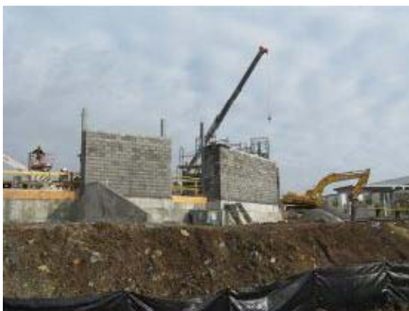
Media Center Steel & CMU
