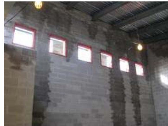
Metal Roof Deck
