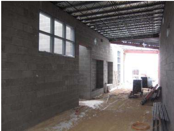
Academic Bldg. Main Corridor
