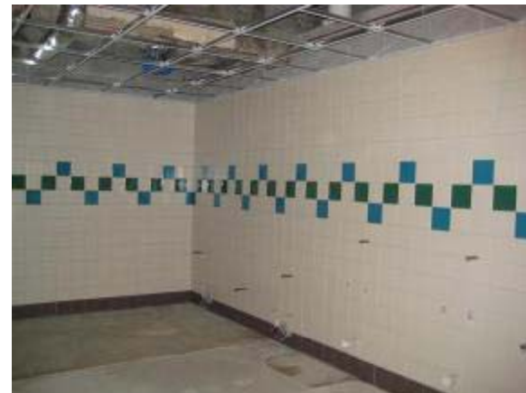
Tile in Boys' Restroom
