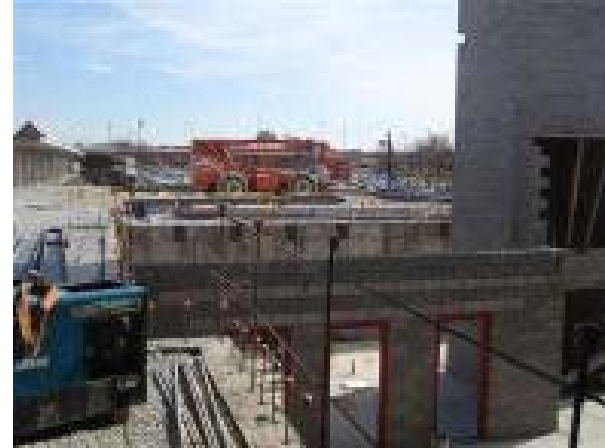
Block Work & Steel -- Gym
