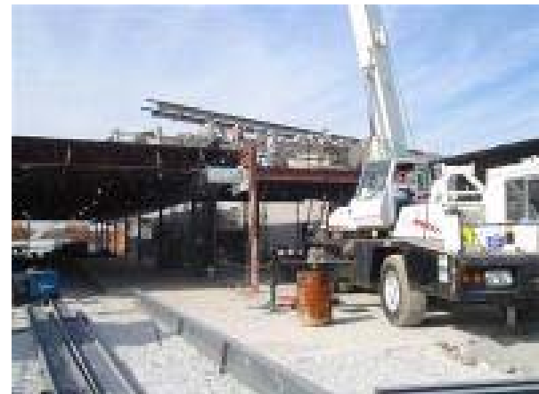
Structural Steel -- Courtyard
