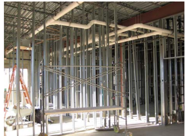
Admin. Area Framing
