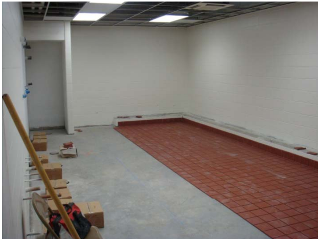
Locker Room Tile Installation
