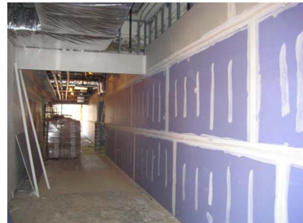
New Drywall in Existing Corridor
