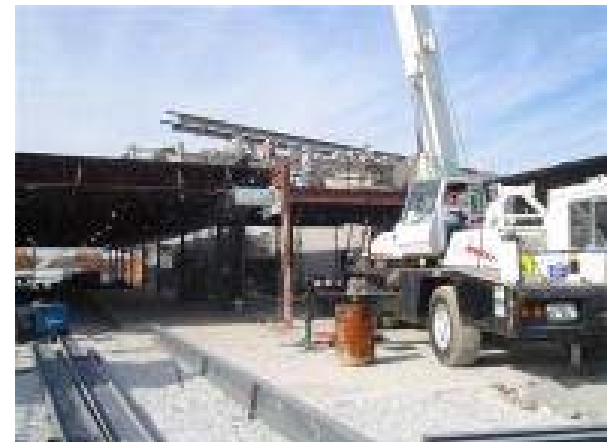
Structural Steel -- Courtyard
