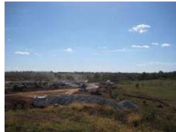
View of Site – West Side
