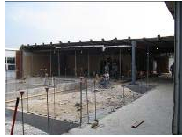
Courtyard Infill – Future Tech Lab
