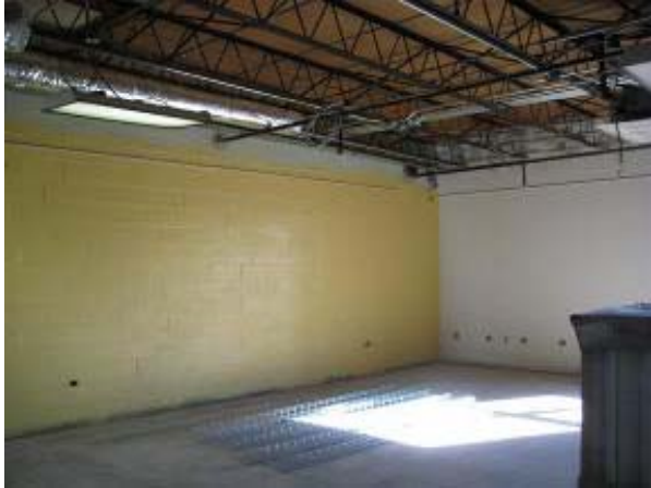
Existing Classroom -- Paint
