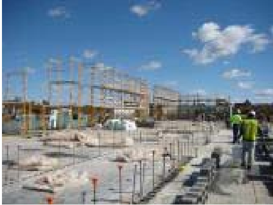
Classroom Bldg. ICF Upper Wall Framework
