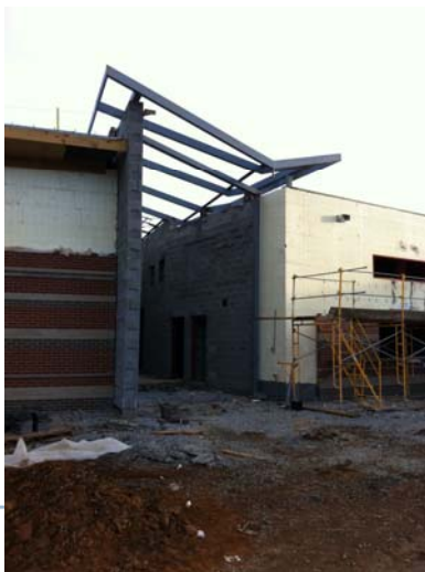
Structural Steel Being Installed
