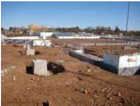
Classroom Bldg. Entry & Foundations
