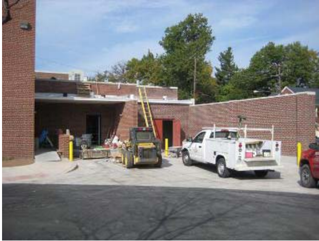
Loading Dock Renovation
