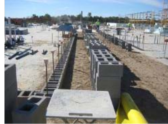
Classroom Bldg. Main Corridor
