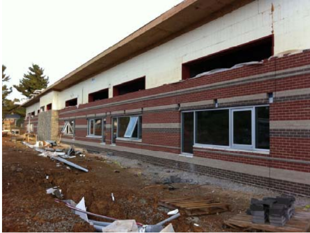
West Wing Windows Being Installed
