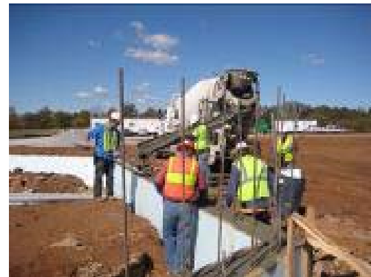
Classroom Bldg. ICF Base Course
