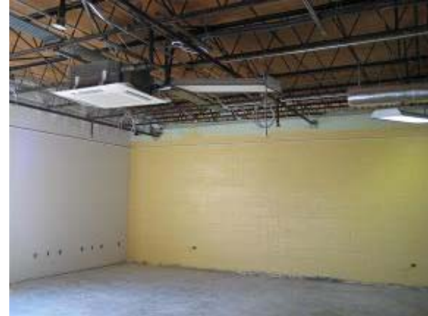
Installation of HVAC Units
