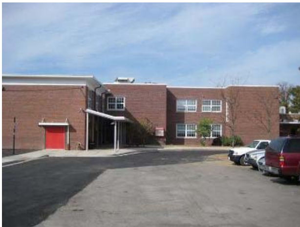
Cassidy Ave. Entrance w/ New Canopy
