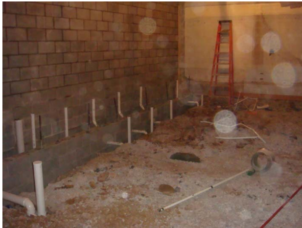
Plumbing Excavation at Shower Room
