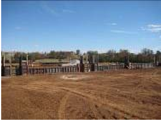
Arena East End Foundation
