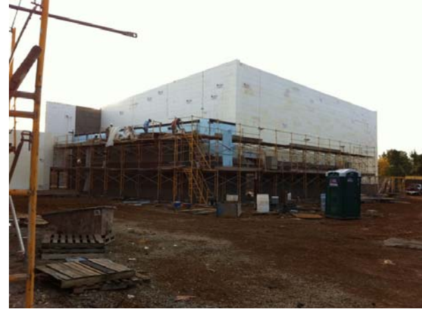
Masonry Install on Gym
