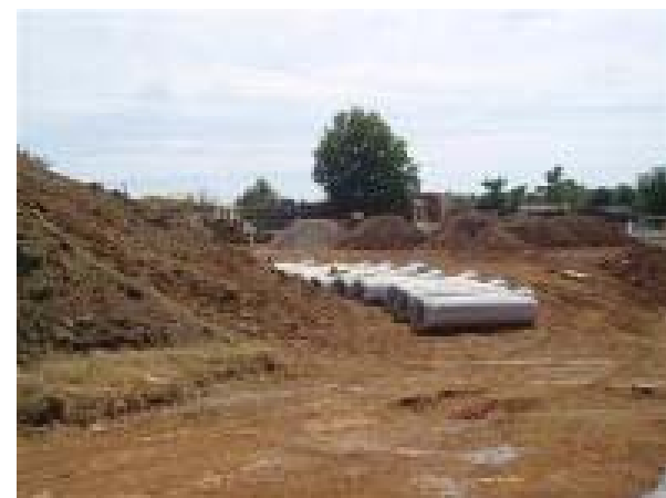
Playing Field Grading Work
