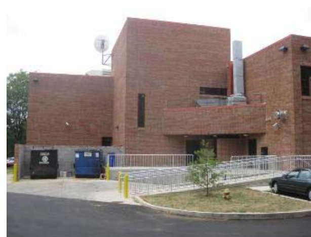
New Kitchen Dock
