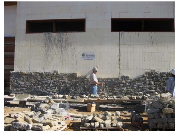
Limestone Being Installed – West Wing
