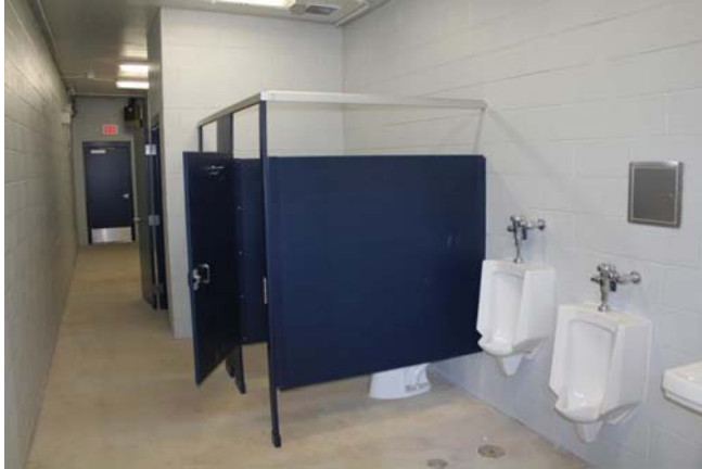
Restroom Building Partitions
