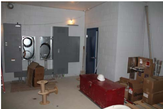
Electrical Work in Sport Support Bldg.
