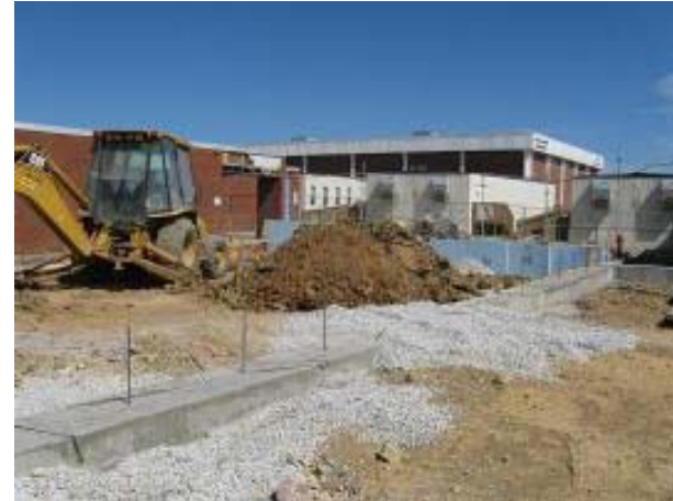
Area A Foundation Work
