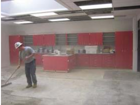
Art Classroom w/ Casework & Skylight
