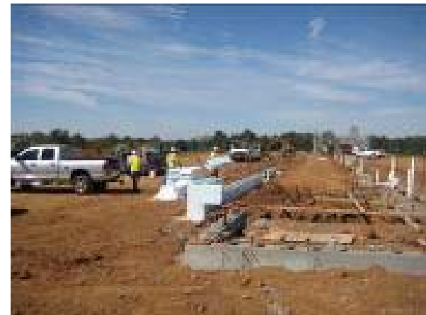
Classroom Bldg. Site – ICF Installation
