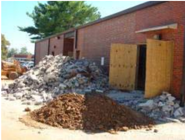
Phase 3 – Exterior Demo
