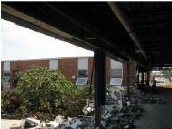
Existing Courtyard Demo
