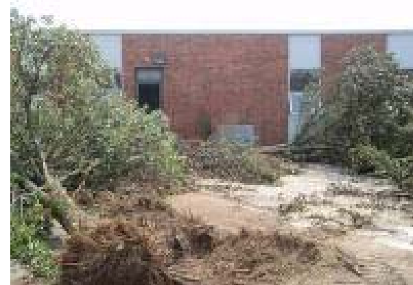
Exterior Grading & Demo
