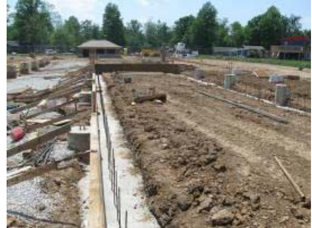
Foundation for Sport Support Bldg.
