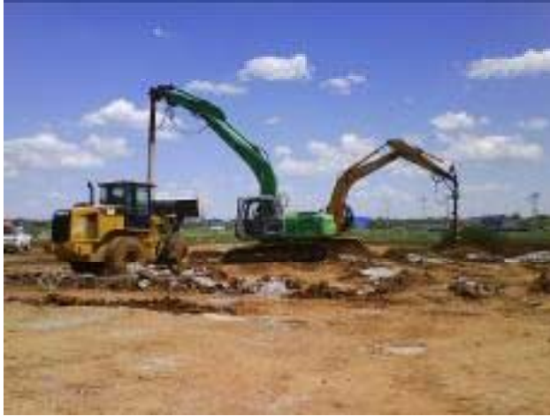
Drilling Pier
