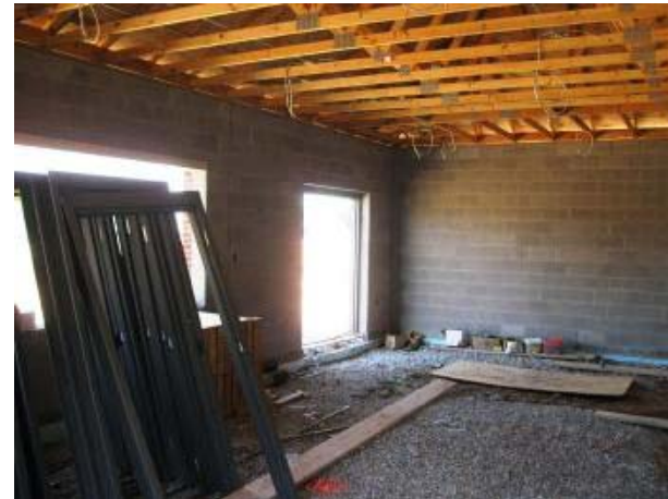
Work Inside Concession Bldg.
