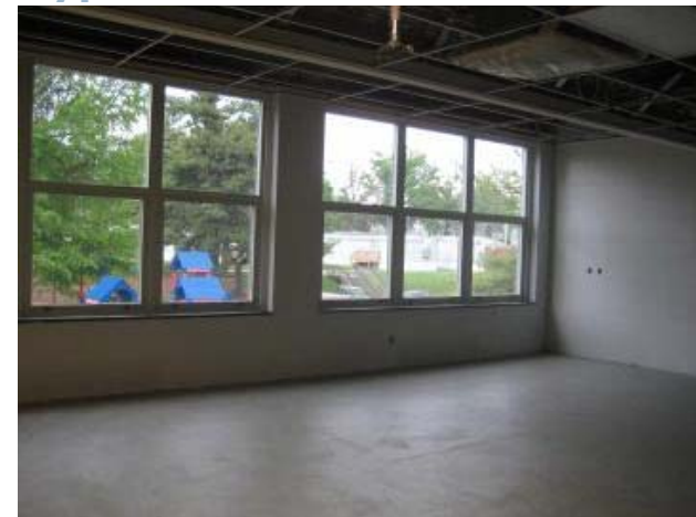
Typical Classroom Renovation
