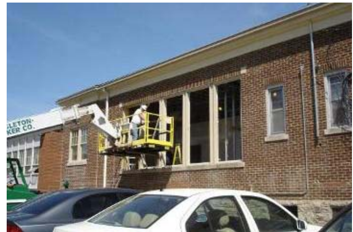
New Window Installation
