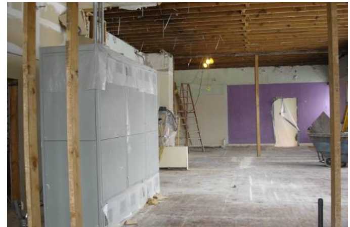
Office Area Demo
