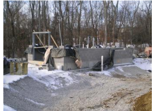
Press Box Masonry Const.
