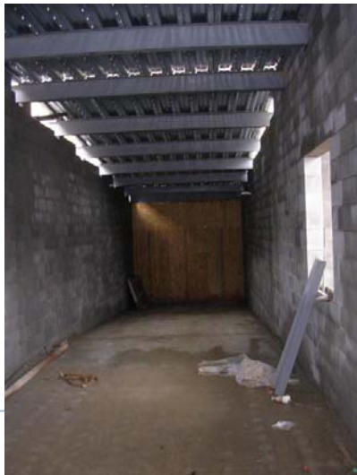
2 nd Floor Framing & Decking
