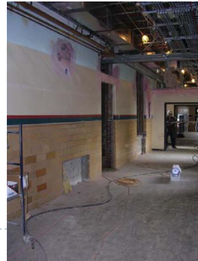
Plastering in Existing Bldg.
