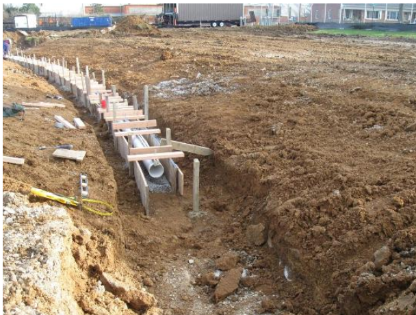
Track Slot Drain Construction
