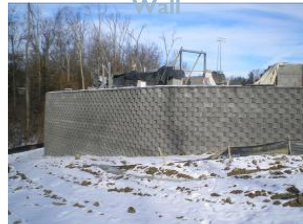
Completed Keystone Retaining Wall
