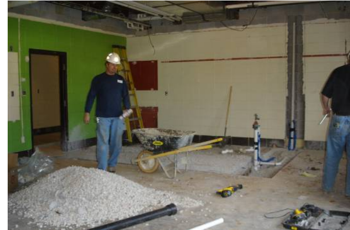
Art Room – Plumbing Rough-in
