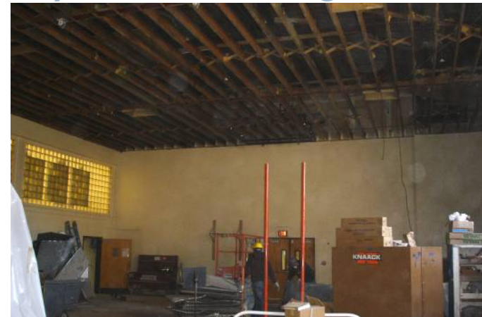
Gym – Plaster Ceiling Removed
