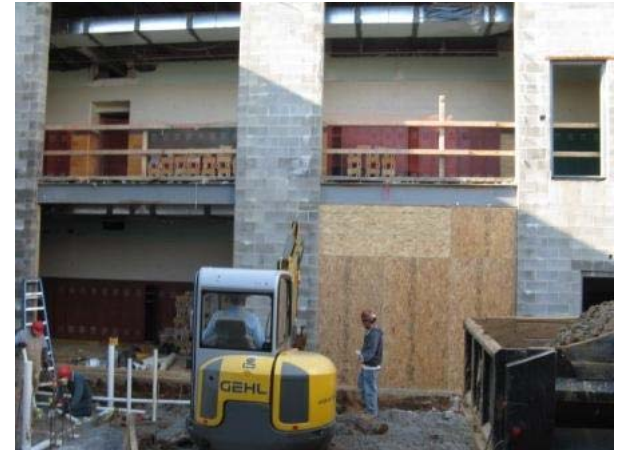
Wall Between Existing & New Facility
