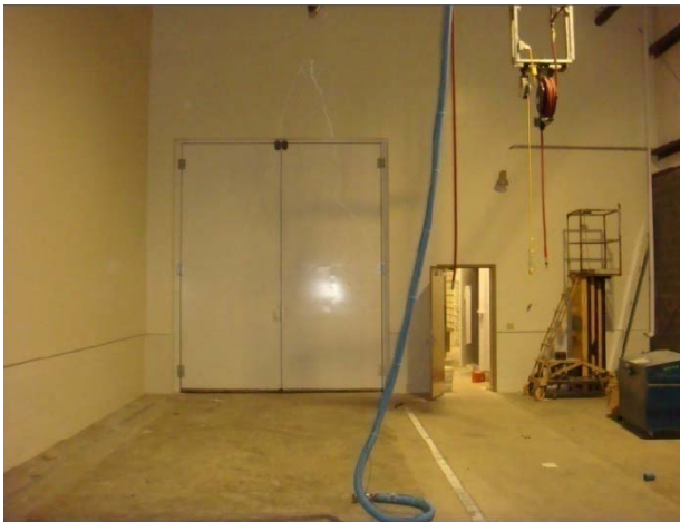
Paint Booth Entrance
