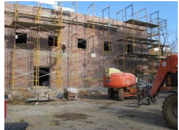
New Brick Walls
