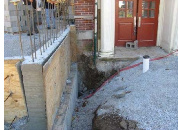
Footers Being Completed
