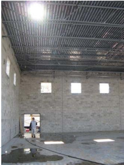
Kitchen & Cafeteria Ready for Slab
